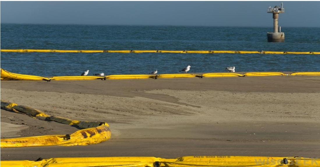
Figure 4. **Cleanup after an oil spill off the coast of Californian. The oils spill skirts border the spill so it does not affect the marine life.**
